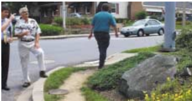
Missing sidewalk near Falls Road Light Rail
