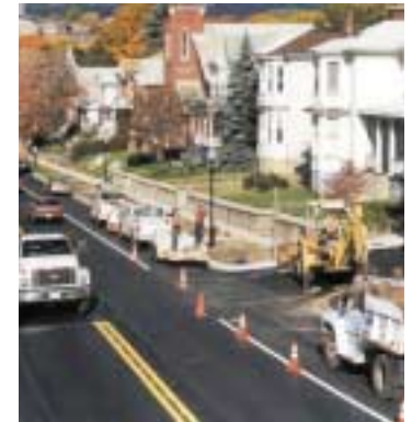
Construction underway in Frostburg.
