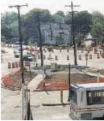
Mt. Rainier roundabout under construction.
