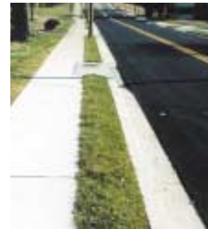
Straight Curb & Gutter, Cecilton, MD
