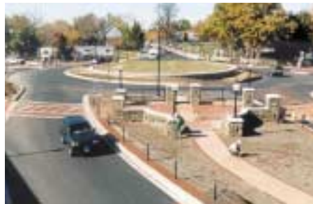
Roundabout, West Street at Taylor Avenue in Annapolis, MD.
